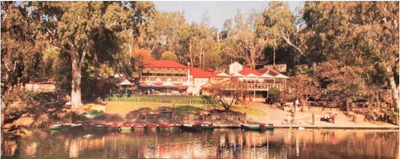
Studley Park Boathouse, by the Yarra River
